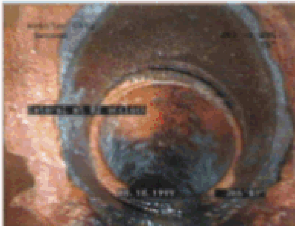
IMAGE: 35_20a, TAPE #: 6, 01:40:20 lateral at 02 o'clock
