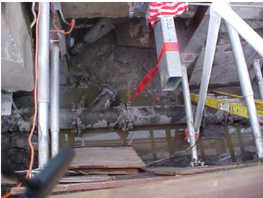
Existing pipe and tunnel entry, Hydro-excavated and shored.
