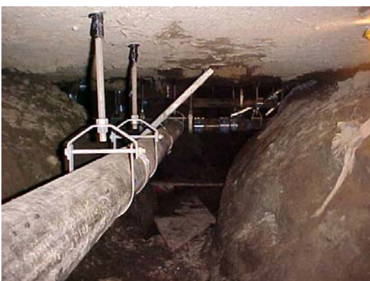
New piping and bracing, installed after tunneling by Bravo crew.
