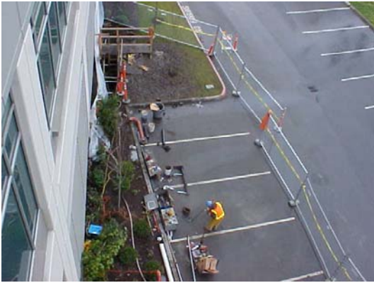
One of the project tunnel entries.
