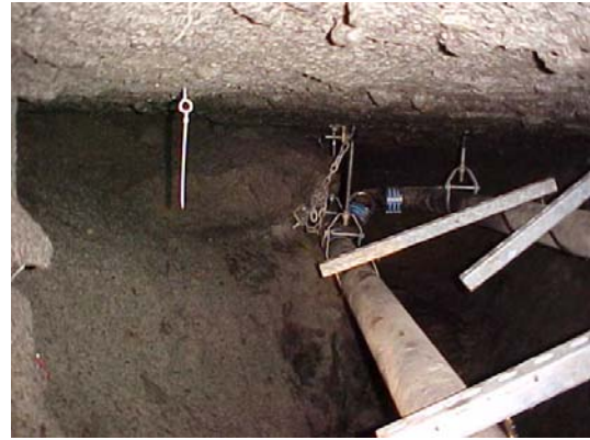
Exposed piping and bracing under building.
