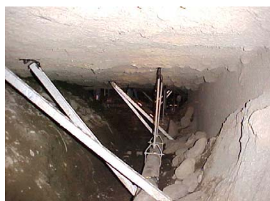
New piping installed after hydro-excavating next to building footer.
