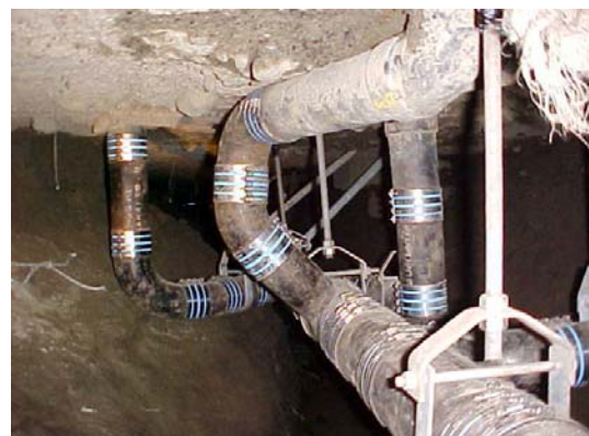
New piping and braces installed after tunneling.
